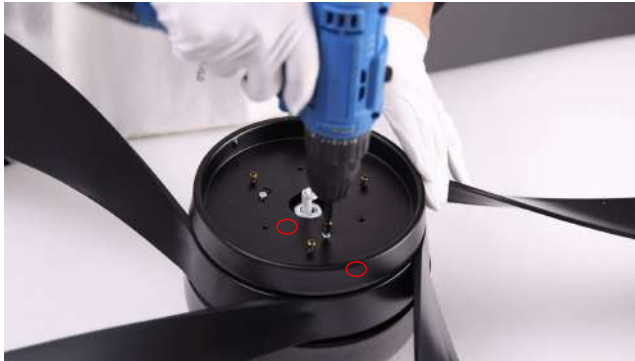
7. Tighten the 3 silver lamp panel screws
