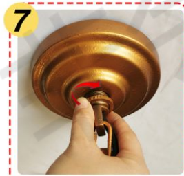
Screw the collar for fixing the canopy.
