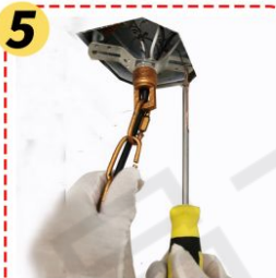
Fix the mounting bracket on the electrical box.
