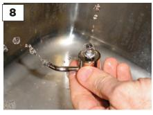
To confirm the top portion is completely clear, hold it as shown and run water through the threaded neck. Repeat steps 6 & 7 and continue to flush until a steady stream of water flows through the threaded neck and out of the spout.
