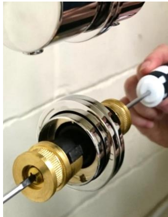
4. Using a Cross-head screwdriver remove the Temperature Handle Bush.
