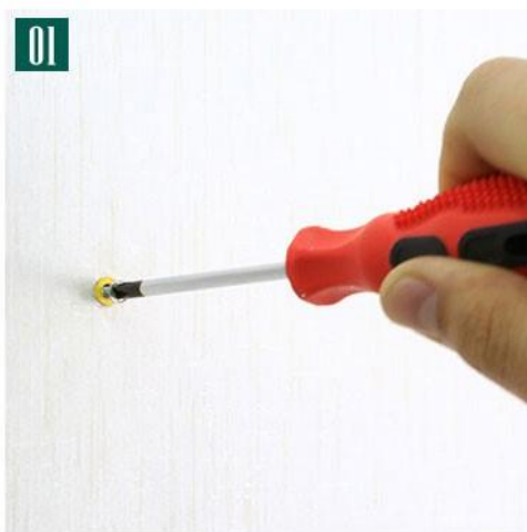
01 Install the expansion screw into the wall
