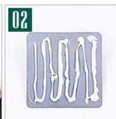
02 Apply a sufficient amount of nail free adhesive evenly on the back
