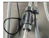
05. Connect the motor to the hose
