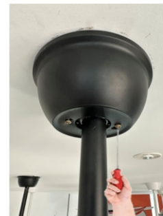
Step 18. Button screw complete
