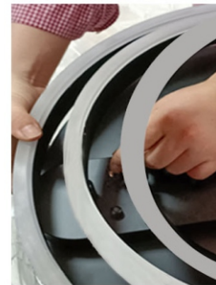
Step 5. Through four The screw button nut will Main body and luminaire installation
