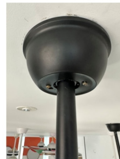
Step 17. Install the bell and horn cover, align the hole and rotate the bell to clamp firmly
