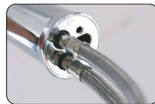
contact hot- cold waterlines and tighten
