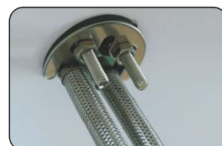
Put nuts on & tighten nuts
