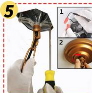
Fix the mounting bracket on the electrical box and connect the wire. Screw the collar for fixing the canopy.
