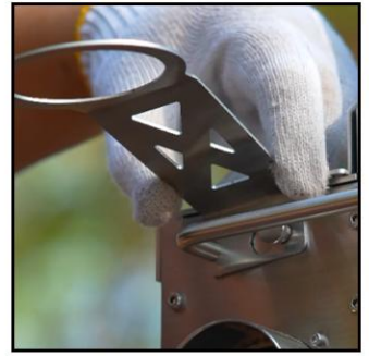
install chimney locking plate
