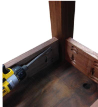
\*Be careful not to over tighten the screws, as this may result in the wood cracking.
