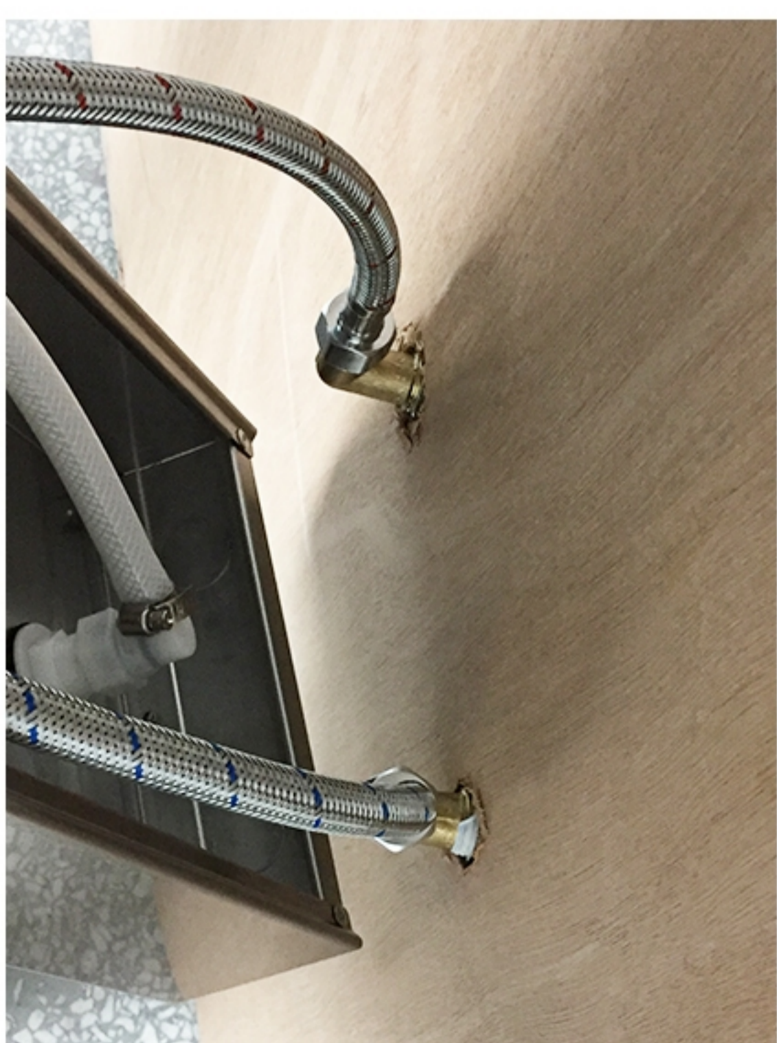
(13). Finish the hose installation.
