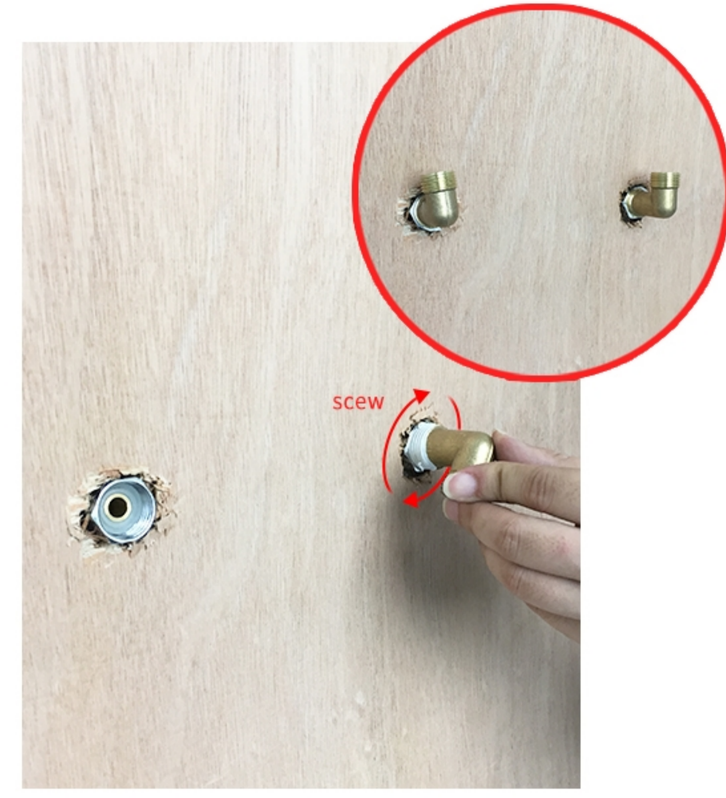
(4). Screw the two connectors.
