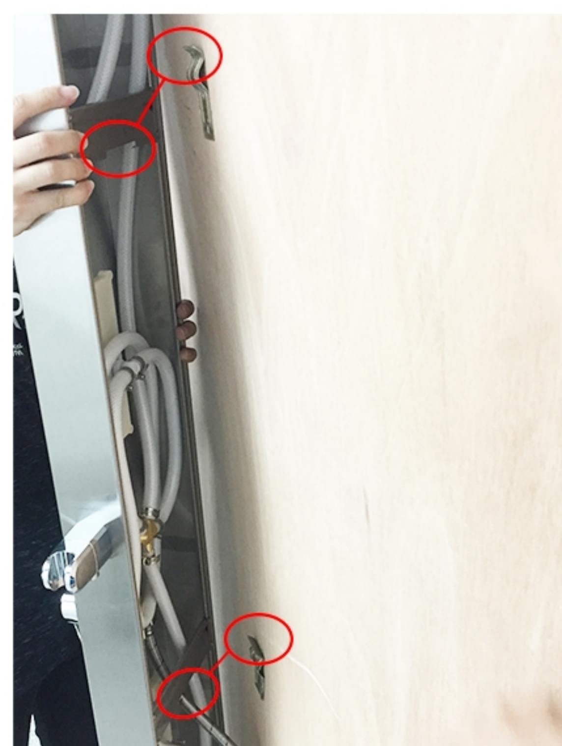
(14). put the shower panel aiming at the top of fixing washer.
