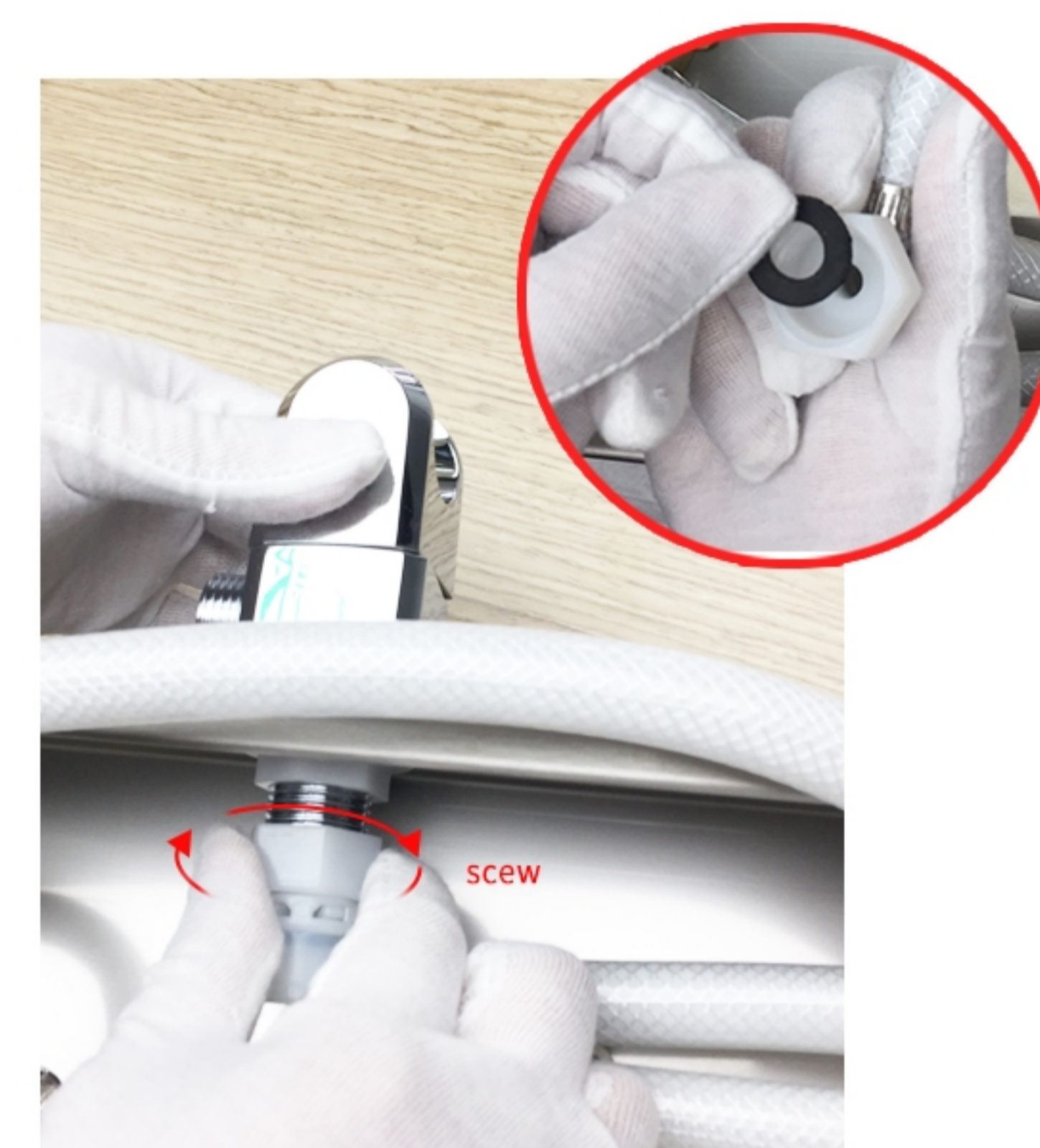
(8) put the gasket into the screw nut and screw them on the base part.
