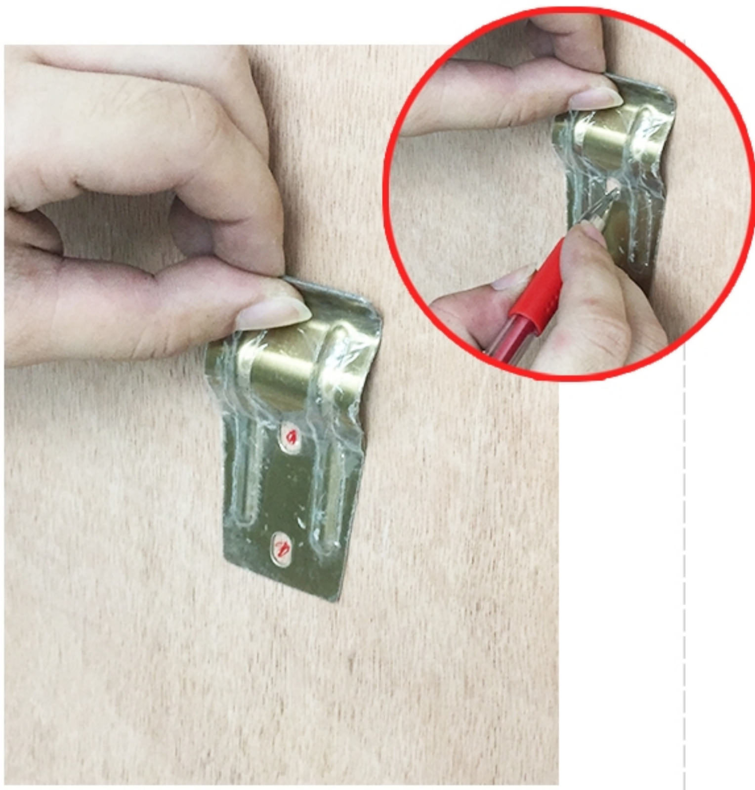
(5). Mark the punching position of fixing washer on the wall.
