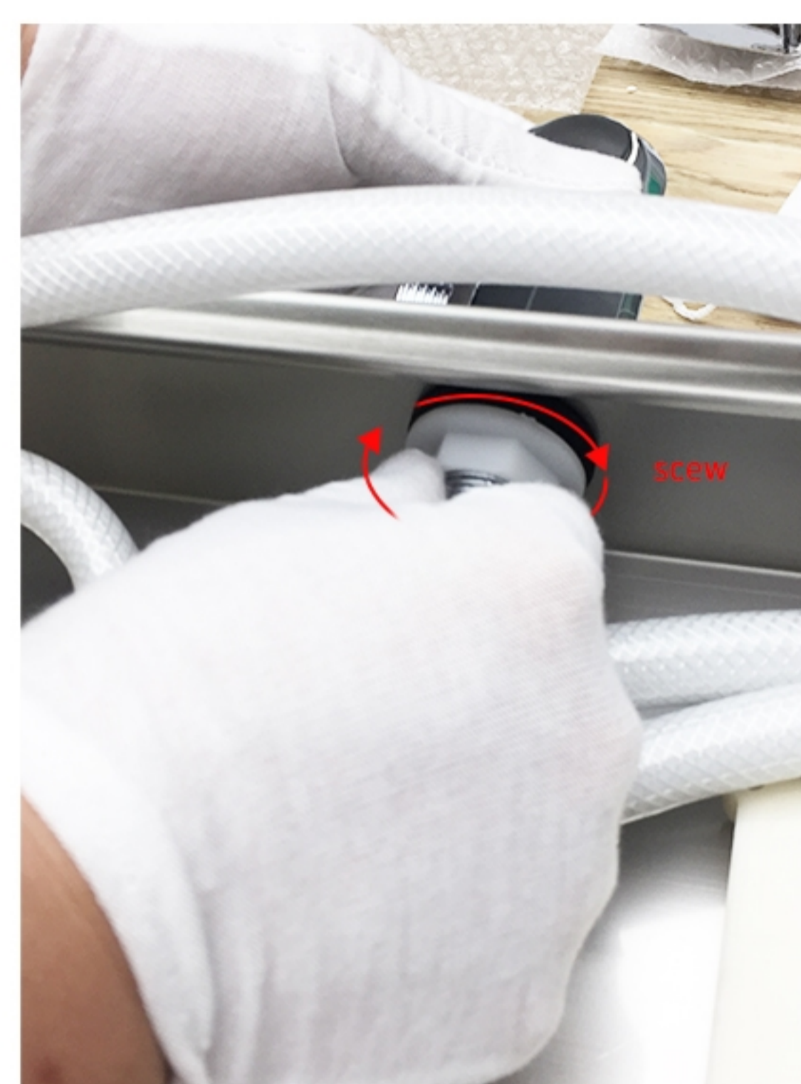
(7) screw the fixing nut and fix the base part
