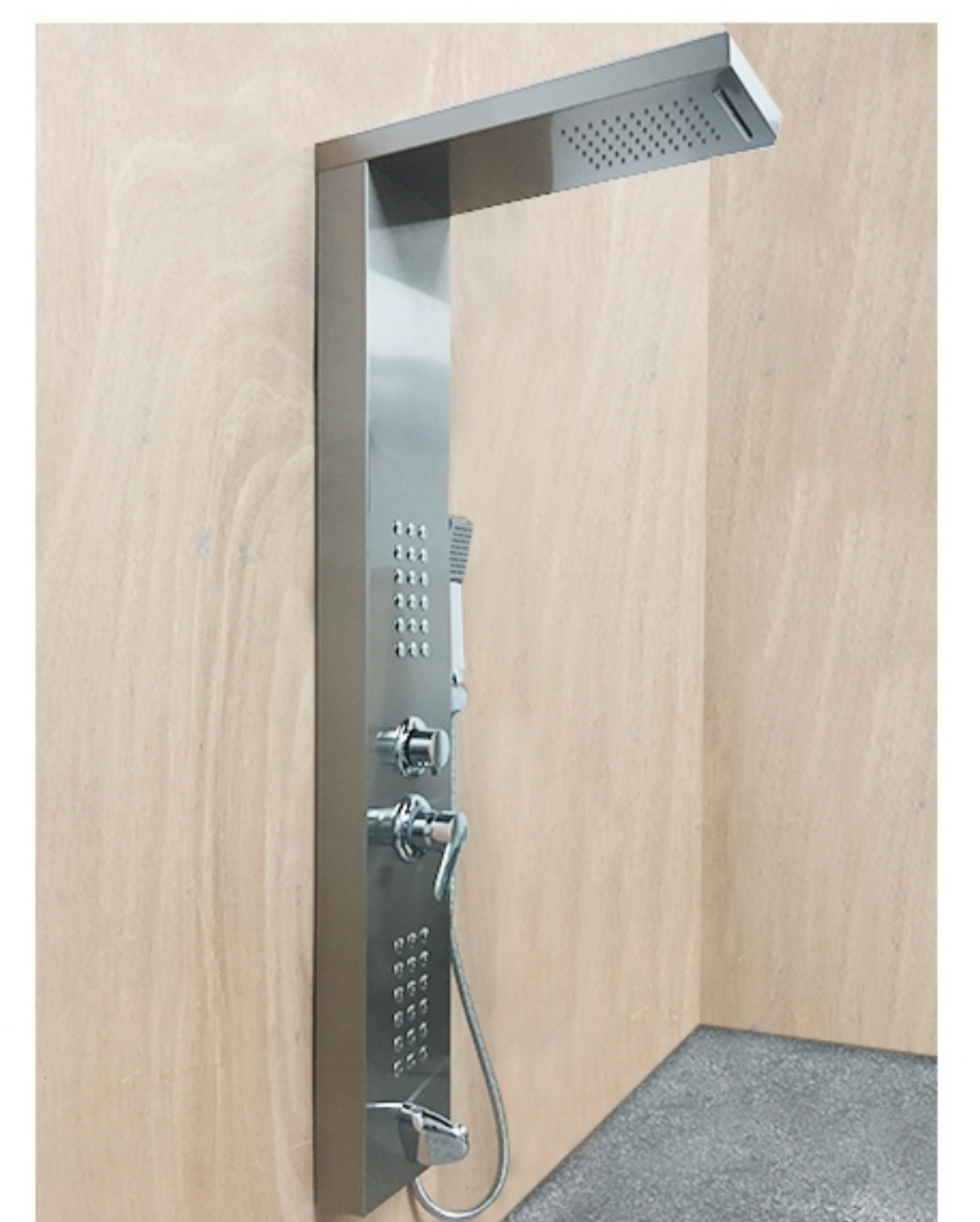
(16). The installation is completed.
