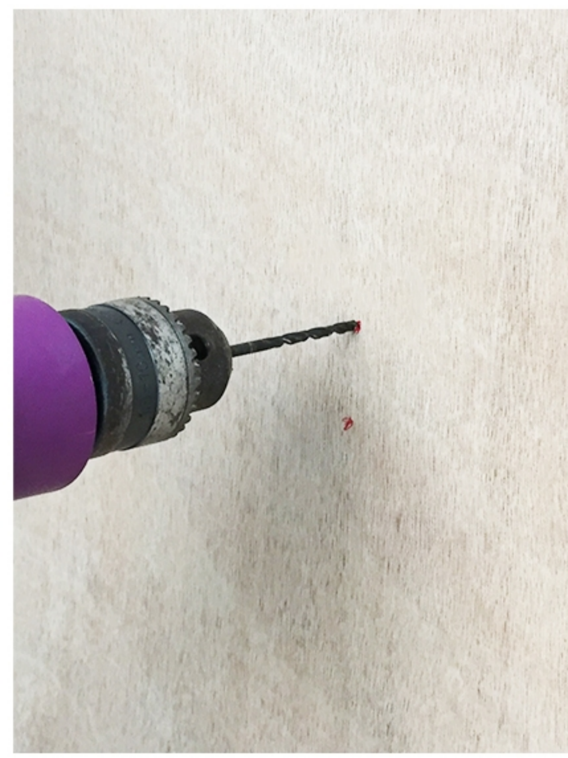
(6). Drill holes at the marked position with an electric drill.
