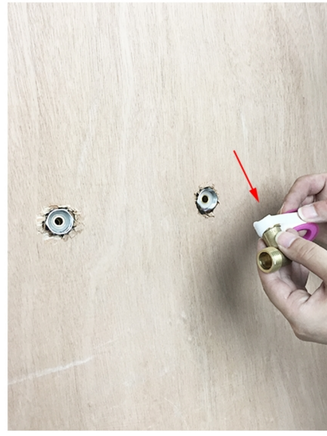
(2). Attach the PTFE tape to the connectors.
