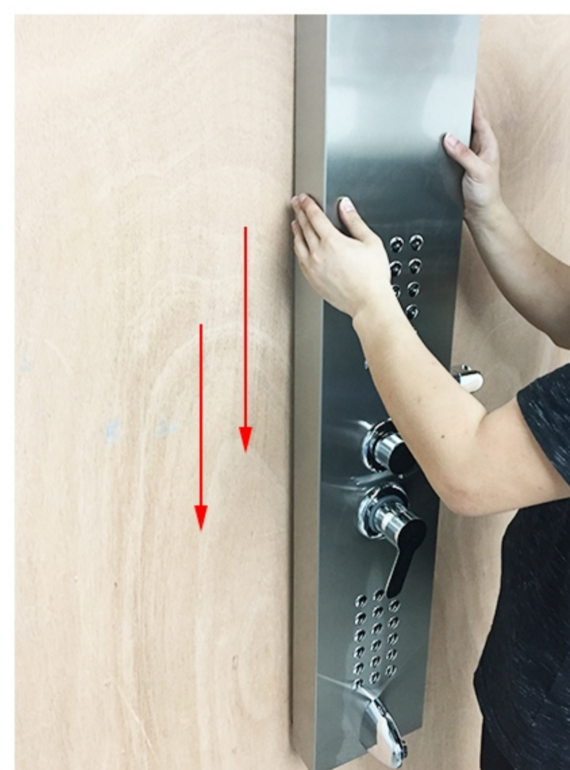
(15). After closing to the wall, pull down the shower panel vertical.
