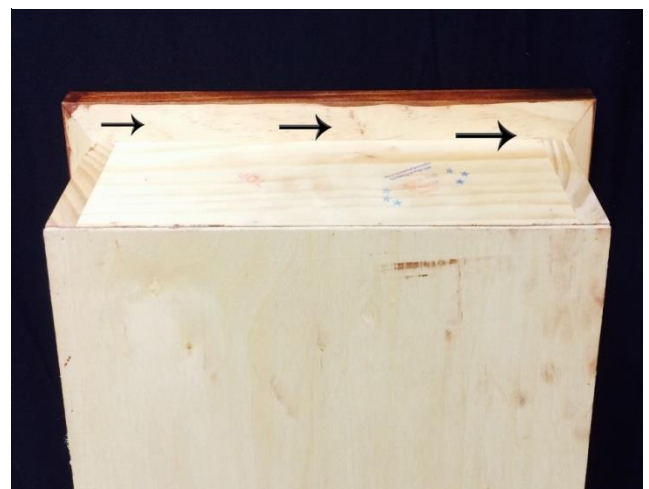
Image 4 Apply Construction Adhesive
