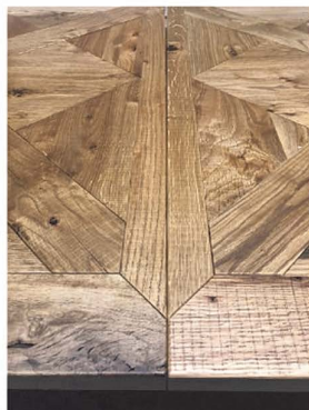
SAW MARKS & VARIANCE BETWEEN PANELS
