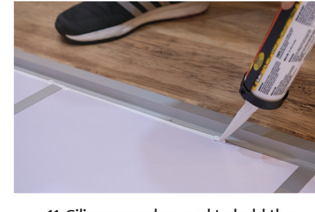
11. Silicone can be used to hold the mirrored panels securely in place
