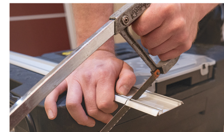
17. Accurately cut the track to size
