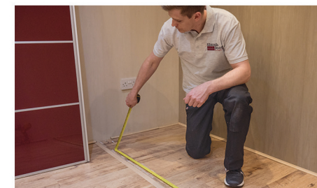
16. Carefully measure the length of track required and make sure the floor is level
