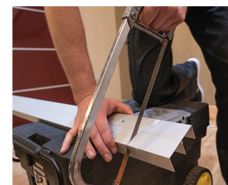
20. Accurately measure and cut the ceiling track to size
