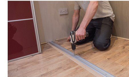
18. Secure the floor track by screwing into the holes provided
