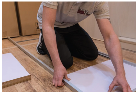
8. Push the bottom panel firmly into the frame
