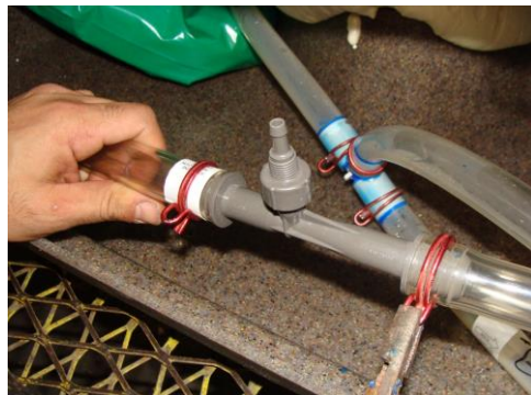
9. Using the pliers, install the hose clamps about center of each barbed end of the ozone injector.
