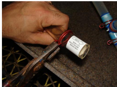
7. Slip hose clamps over each end of the cut hose, it may be necessary to use the pliers to do this.
