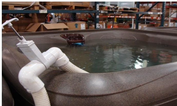
18. Fill the spa with water before connecting electrical.
