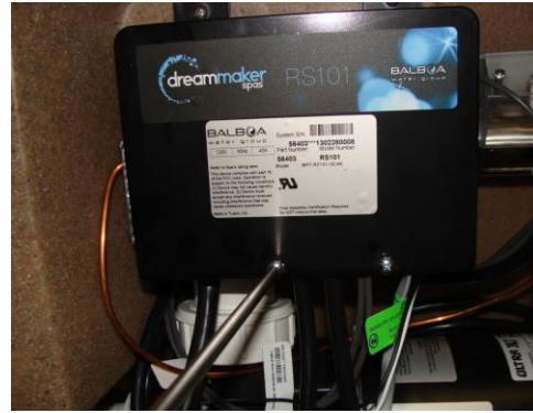
17. Attach the control box cover, and then attach the equipment access door.
