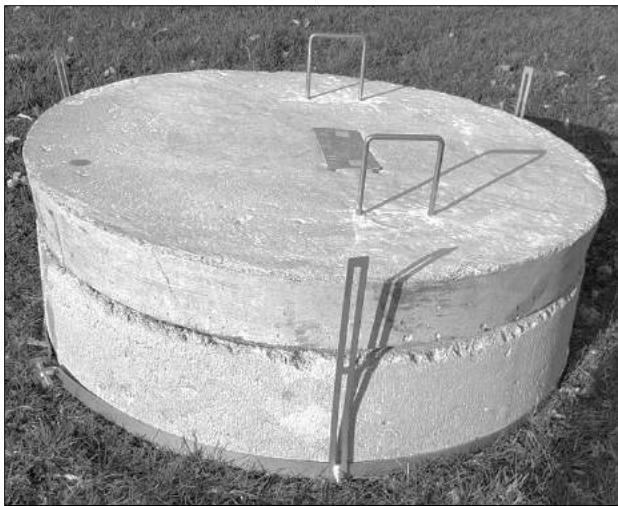
Septic lid with the hoop installed properly.
