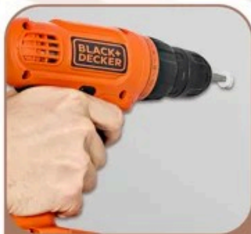
Drill Anchor into Wall
