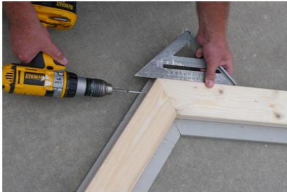
To construct the Rake begin by squaring the rake and fasten with 2 1/2'' screws.
