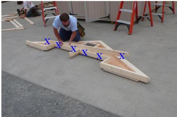
Now install 2x4 brace as shown above, secure with 2 1/2" screws on the X's. Then install gable vent as shown in previous pictures. (refer to #21-#23)
