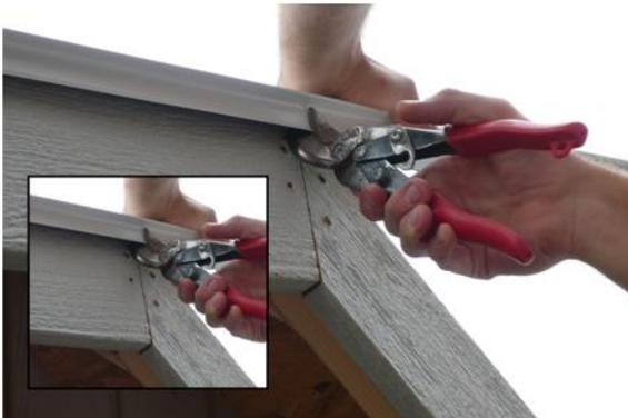
As you secure the drip edge, you will need to snip the drip edge to allow bend along the ridge.
