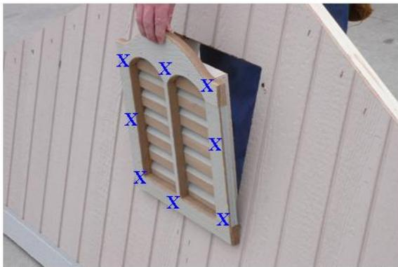
Next install the wooden vent and secure with 1 1/4" screws at each X.
