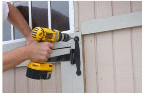
The piece of trim at the top of the double doors will fit behind the door hinge, you will then fasten the trim with a 2 1/2" black headed screw into the hinge through the trim.
