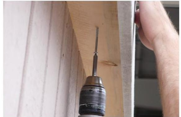
Temporarily fasten the brace to the top plate with a 2 1/2" screw from the outside of the building.
