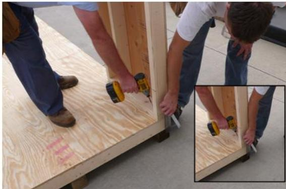
Locate the first wall panel, then set in place. Make sure the wall is flush with the edge of the floor structure, by using an angle. Apply pressure from the outside and secure the wall panel to the floor using 2 1/2" screw.
