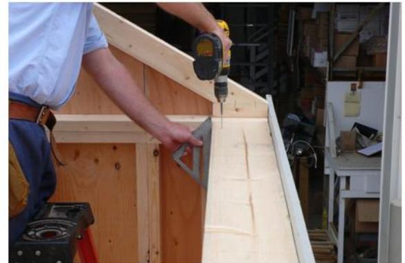
Next find the 2x8 plate, now lay the 2x8 plate making it flush with the 2x4 on the inside of the wall. Fasten the 2x8 to the 2x4 with a 2 1/2" screw.
