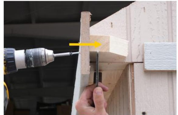
Fasten the trim board with 1 1/4'' screw into rake block.
