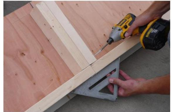
Next you can fasten the bottom of the gable with 2 1/2" screws.
