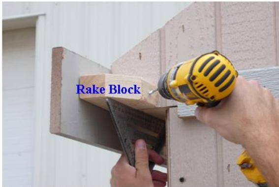
Install small rake block as shown. Fasten with 2 1/2'' screw.
