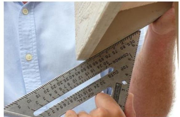
Install outside rake and use angle to make flush with bottom of Fascia.
