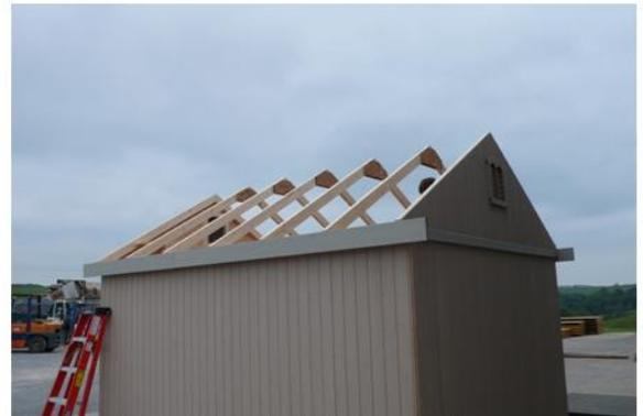
Picture above shows building ready for OSB sheathing.
