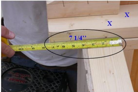
Position the gable by measuring 7 1/4" from the inside of the wall to the end of the gable. Then secure with 2 1/2" screws at each X.
