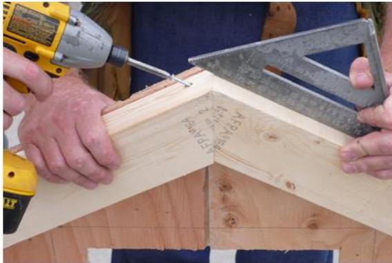
Placing the 2 gable sections together (as shown above), make sure it is square, and then fasten using 2 1/2" screws.
