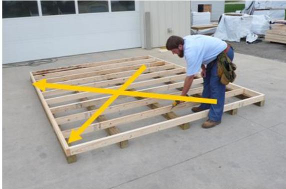
Now place 2x4's, 16" on center, on top of the 4x4's, place 2 1/2" screws in each of the 4 corners. Measure from corner to corner to make sure it is square. Now you can fasten each 2x4 to the 4x4's with 2 1/2" screws.
