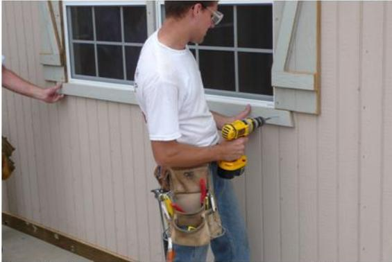
Install trim on the bottom of windows and fasten with 1 1/4" screws.
