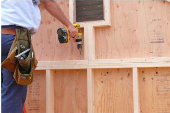
The gable can now be fastened to the top of the wall with 2 1/2" screws.
