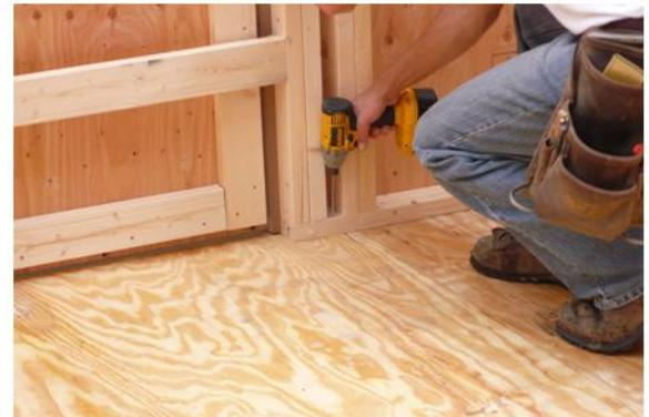
To completely secure, fasten with 2 1/2'' screw into 2x4 through the floor.
