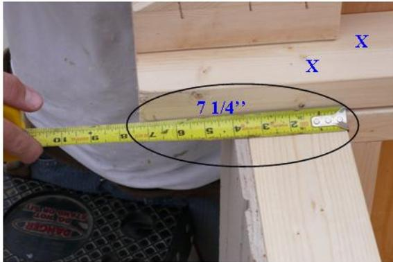
Position the gable measuring 7 1/4" from the inside of the wall to the end of the gable. Then secure with 2 1/2" screws at the X's.
