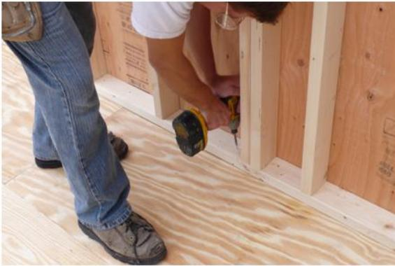
...to completely secure the wall panel to the floor place 2 1/2'' screws 16'' on center
