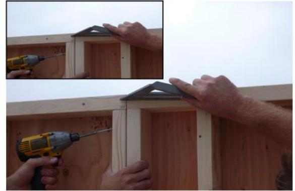
Where each panel meets another, use an angle and make sure 2x4's are flush and fasten with 2 1/2'' screw.
