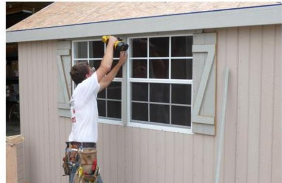
To install the window trim, secure with 1 1/4" screws.
