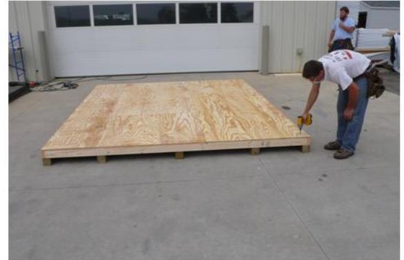
Next set sheet in place and make sure sheathing is flush on both sides. Secure in place by driving 1 1/4" screws through the sheathing into the 2x4s every 8".
