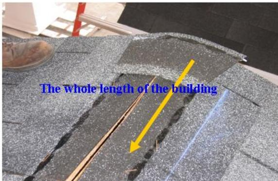
Cut Ridge cap in shape as shown in picture and start to place cap on top of building.
