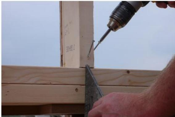
On the Gable end, locate the center of the window opening, here you will want to secure the 2x4 with 2 1/2" screws as shown above.
