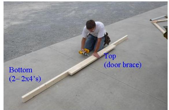
Now you need to construct your temporary brace, you will use this to brace the building before setting the trusses. You will need (2) 2x4's, that will later be used for collar ties, and your top piece will be the door brace that was used in shipping
