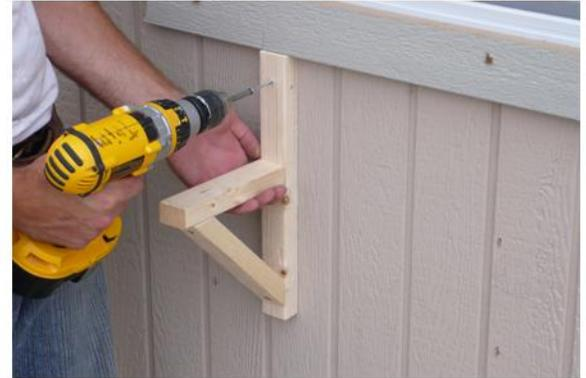
To install flower boxes, begin by installing the mounts. Fasten with 2 1/2" screws on top and Bottom.
