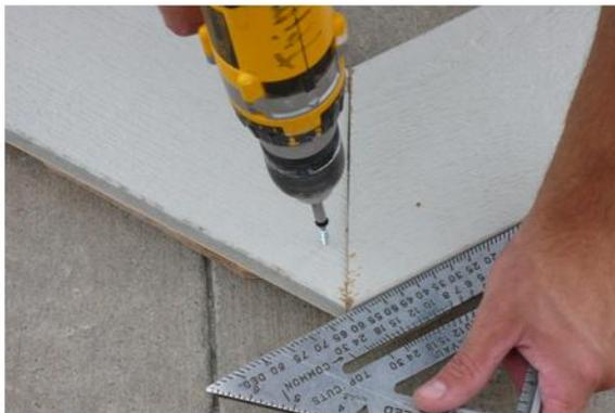
Square peak of 1x6 trim for Rake and fasten onto 2x4 Rake with 1 1/4'' screws.
