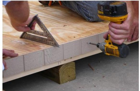
Place the small piece of duratemp siding (this is the piece we set aside to use underneath of the door) below door opening and use angle to make flush. Fasten with 1 1/4" screws approximately 8" on center.
