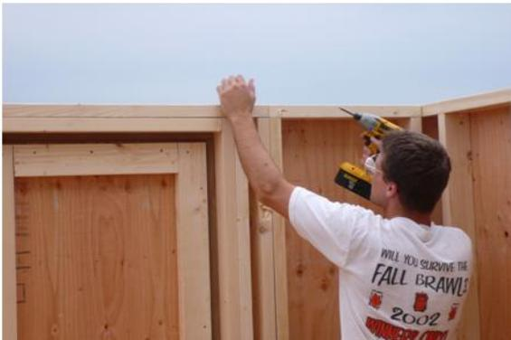
As you did with wall panels, use an angle to make sure 2x4's are flush and fasten with 2 1/2'' screw.
