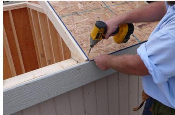
Now you are ready to install the roof sheeting. Start with the bottom sheets. You will fasten each sheet on the outside edge with 1 1/4" screws.
