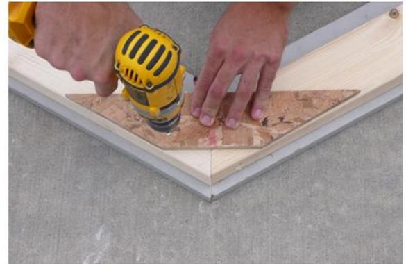
Set truss Gusset in place and fasten with (8) 1 1/4'' black headed screws.
