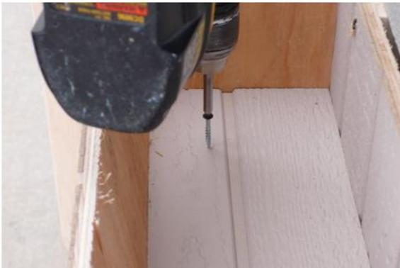
Fasten with 1 1/4" black headed screws into the mount as well.
