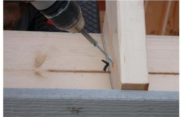
Secure each truss with 2 1/2" screws. Going into the side of truss secure one screw on each side.
