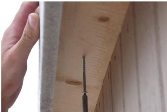
Then fasten from the bottom as well. Secure from bottom of 2x8 top plate with 2 1/2" screws.
