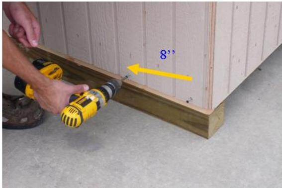
Fasten wall panels from the outside at the bottom with 1 1/4" screws every 8".
