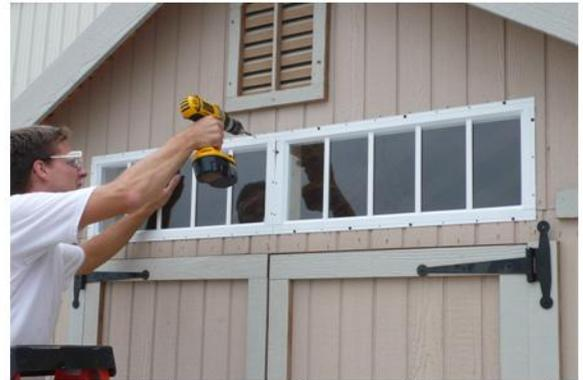
...secure with 3 screws at the top and 3 screws at the bottom, per section.
