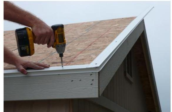
Next your are going to install the drip edge. This will be fasten with 1 1/4" screws.
