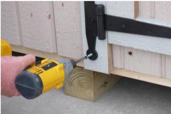
Fasten the bottom door hinges with 2 1/4" black headed screws.
