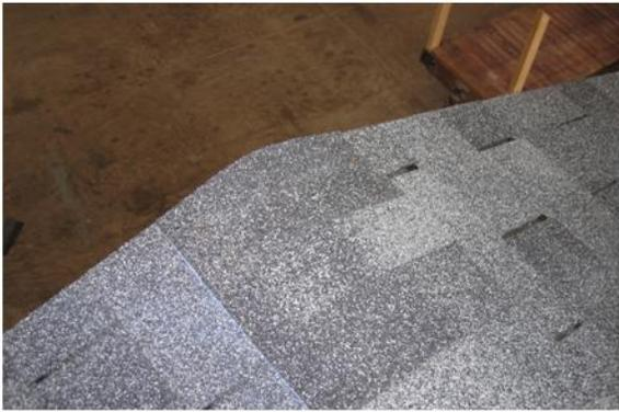
Continue to edge of the building. You can finish with a smaller cap with an adhesion strip.
