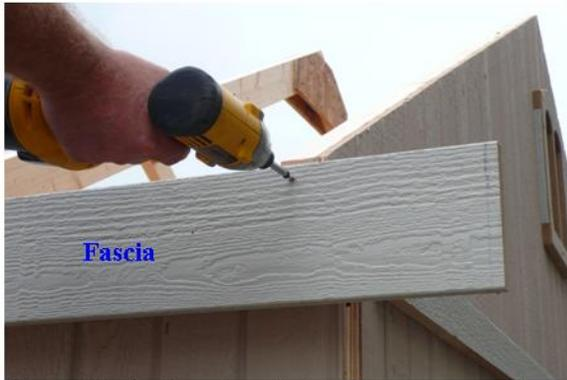
Secure the 1x6 Fascia with 1 1/4" screws at each truss.
