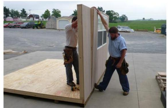
Position next panel in place and fasten to sheathing along the bottom with 2 1/2" screws...
