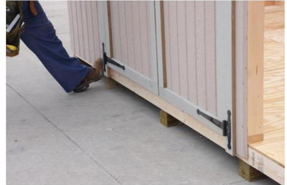
Door panel will attach just as a wall panel, apply pressure on the outside and fasten with 2 1/2'' screws on the inside.
