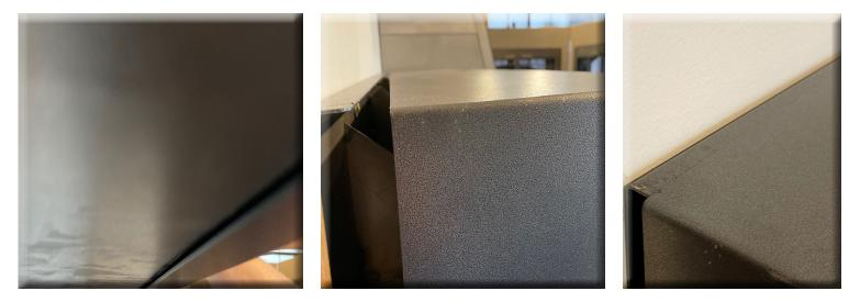
8. Carefully and gently apply firm pressure to all area of mantel cap, assuring that it is locked in tight and flush with wall.
