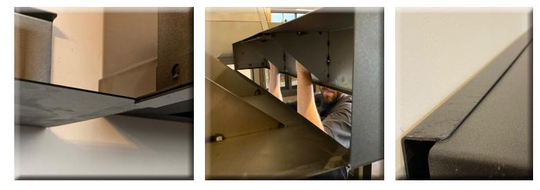
7. Using two people (preferably) slowly and gently slide the mantel cap in place onto the base as shown .Mantel cap should get snugger feeling as it gets close to flushing into wall.
