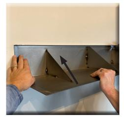
**4.** Using two people (preferably) hold base up to line and use screws to mount base to wall. Be careful to assure you are screwing into the center of studs or other solid backing system.
