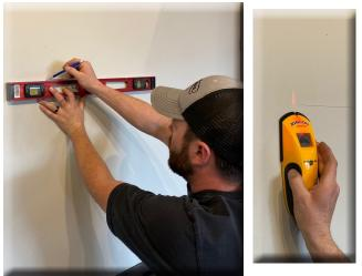
**3.** Mark where mantel will be installed and use level to mark a line across wall. You may also want to use a stud finder to identify stud locations to screw to.
