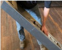
2. If panels have a bow in them, which can happen in the freight process, they are generally easy to adjust back. Place bowed area across leg as shown and give mild pressure to both sides to conform bowed area back into position. You may have to do this several times with increasing amounts of pressure to get bow out of steel. Do this to both the base and the mantel cap
