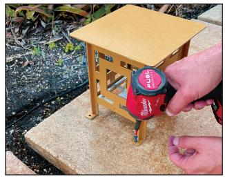
Attach to Deck, depending on your serface, wood, concrete, pavers etc. Any Hardware Store can direct you to the proper fastener type.
