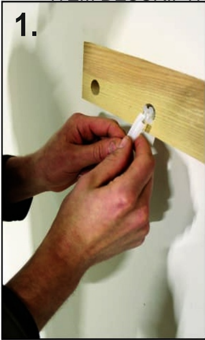
1. Insert the plastic dry wall anchor inside the hole drilled into the wall through the wooden support
