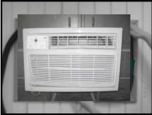
1. Install the 1" x 1½" x 84" long stuffer-seal between the wall-sleeve and the unit. A flat-bladed screwdriver or putty knife is recommended.
