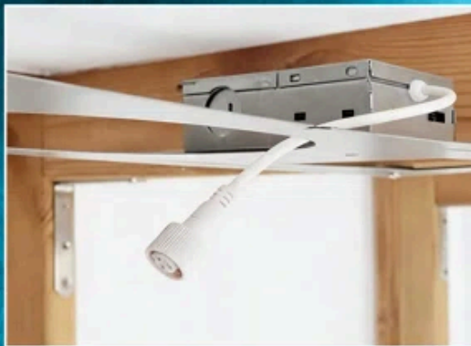
2. A junction box is pre-reserved on the top for wiring connections
