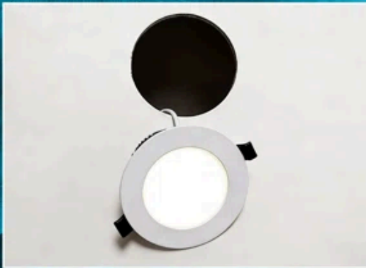
4. After drilling and wiring connections, embed the light
