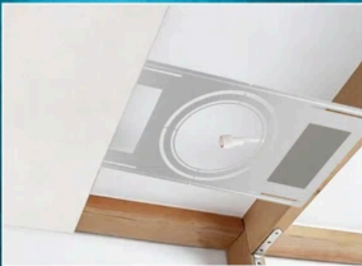
3. Seal the ceiling with gypsum board
