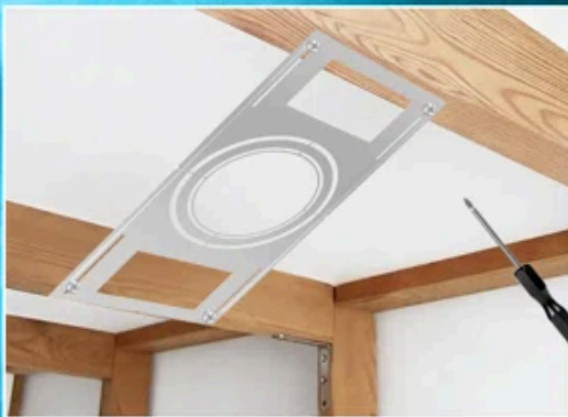
1. Securely fasten the mounting plate with screws
