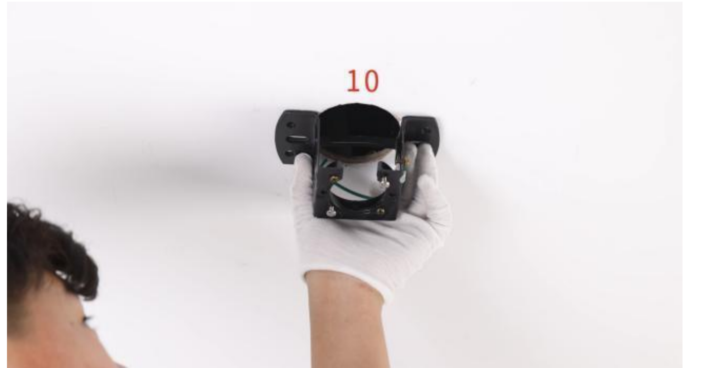
28. Install the ceiling bracket with four self tapping screws
