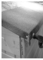
2 Starting at the back lower edge (the eaves) place one piece from the left side to the right side of the building. An overhang of approximately 45mm should be allowed on each of the 3 sides although the felt will overhang one side by more than this.
