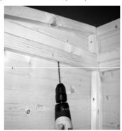
3 Drill through the end panel from below (not the triangular panel) and fix using 3x60mm screws.
