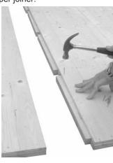
4 Once all frameworks are fitted between floor joists slide the other floor on top of framework and secure again using 3 x 40mm nails per joiner.
