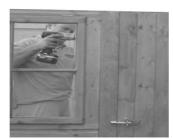
7 Place the 150mm door block on the inside of the door below the horizontal bar in the centre against the opening edge . Fix with 2 60mm screws. The pad bolt must fix to this block and the centre bar from the outside
