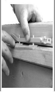
5 Fit the Casement Stay on the window using 2x25mm screws.
