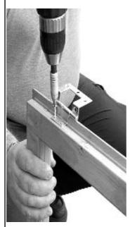
2 Place the window into the aperture. Secure the window to the panel using 3 x 25mm screws per hinge, again through the predrilled holes in the hinge. Repeat for other hinge.
