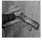
Place padbolt housing in position to accommodate the padbolt. Secure using 2x 25 mm screws using the round holes only.
