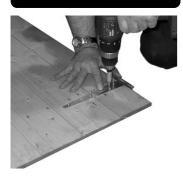
1 Place the door on a flat level surface outside of door facing up. Check which side of the door the hinges are to be fitted, which is the edge with the groove. The hinges are to be fitted on to the boarding which covers each horizontal door bracing.
