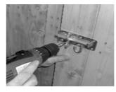
8 Place the padbolt in position on the outside of the right hand door 'D' directly over the central horizontal brace. Ensure the edge is flush with the upright edge. Secure using 4x 25 mm screws using the round holes only
