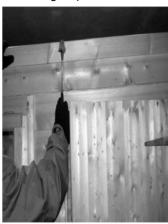
7 Carefully trim off excess felt with cutting knife against the edge of the facia board.
