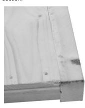
3 Place floors on your firm level base. Take the 5 pieces of floor joiners 34x46x345mm and place between each floor joist. Nail half of the widest part to the floor using 3 x 40mm nails per joiner.
