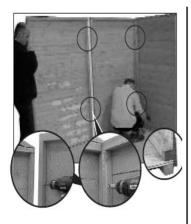
2 Drill 2 holes, one to the top and one to the bottom. Do not drill into adjacent panels. Secure the panels together using 2 x 60mm screws per panel.
