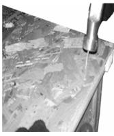
4 Nail into top of framework using 4 x 40mm nails per side and 8 x 40mm nails along the back. Nail into lower support bearer using 3 x 40mm nails...
