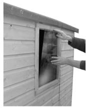
1 Place the glazing material in the window aperture of the window frame.
