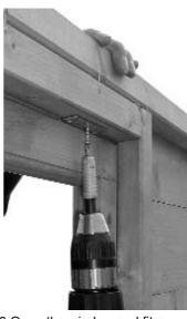
3 Open the window and fit a further 2 x 25mm screws per hinge next to the one already fitted in Step 1. Repeat.
