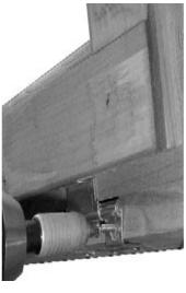
4 Fitting the Casement Stay. Place the casement stay centrally on the inside of the window. Place the 2 pins under the casement stay. Position so that it is not resting on the framework of the panel and not so high that the pins are of no use.
