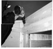
1 Position rectangular pent panel ensuring that the panel is positioned evenly and flush along the top edge of the front panel and with each side. Drill 4 holes from above through the pent panel, either side of the centre upright. Do not drill into the panels below. Secure into position using 4 x 60mm screws.
