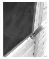
2 Place four strips of beading around the edge and nail into position using 2 x 15mm panel pins per piece of beading. The beading may need to be swapped around to get the best fit. The beading may need to be bent and allowed to 'ping' into place. It may well be a tight fit. Repeat for all widow apertures.
