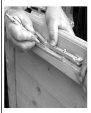
7 Secure into position using 4x 25mm screws - 2 in each pin.
