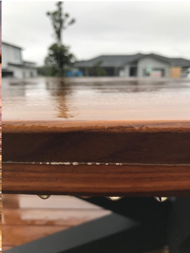
GLUE LINE AT LAMINATION
