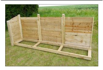
Remove the blocks from beneath the 3<sup>rd</sup> panel and then slide the base into position as shown.
