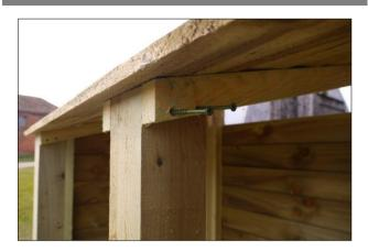
With the centre post lined up with the guide marks on the base, locate the top of the post between the central roof battens, flush with the batten ends, and secure in place with 2 of the shorter green screws.
