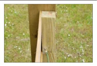
Attach the panel to the post by screwing through the batten using a short green screw as before.
