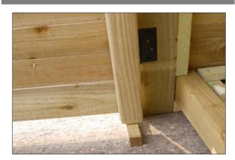
Place a spacer block at the front of the log store adjacent to the front end post and rest the hinge side of the appropriate door on the block, aligning it vertically and horizontally for a good fit. Now use four of the supplied black hinge screws to affix the hinge to the post.
