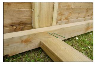
Using more of the longer green screws now attach the base to the rear posts as shown.
