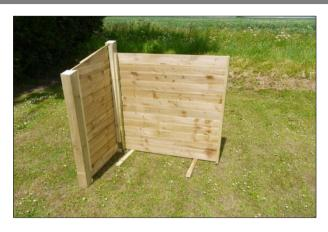
Arrange the 2 spacer blocks on the ground (the orientation is not critical), adjacent to the end panel as shown in the photo above. Now place a back panel on the blocks, at 90° to the end panel, aligning the 2 panels ready for fixing.
