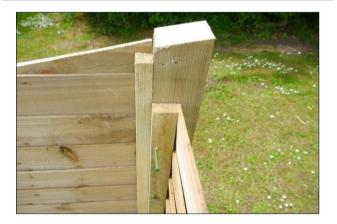
Using the shorter green screws provided, attach the batten on the back panel to the post of the end panel through the pre-drilled holes, ensuring that the batten remains vertically aligned to the post.
