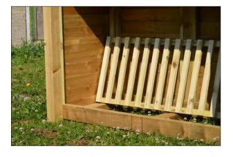
Sit the lattice in the store so that it is leaning against the back panel as shown above, so that you have enough clearance to attach the front posts as shown in the next step.
