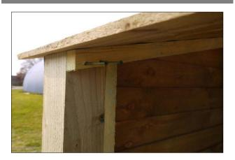
Carefully place the roof on top of the end panel posts ensuring that the batten ends sit flush with the posts as shown. Now attach the roof to each end panel post with shorter green screws.
