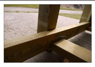
Check the positioning of the post within the guide marks once again before securing the bottom of the centre post with 2 more of the longer green screws. Repeat steps 16 - 18 for the remaining centre post.
