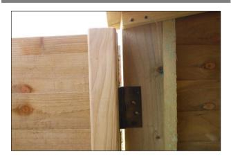
Align the top hinge in place, ensuring that the gap between the door and post is consistent at top and bottom.
