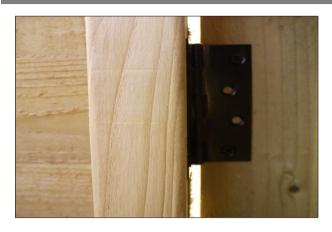
Secure the top hinge in place using more of the black hinge screws. Repeat steps 20 - 22 for any further doors as required.
