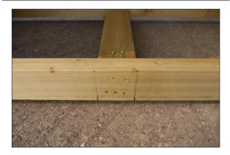
Locate the pencil guide marks on the front face of the base. This is where the centre posts will be fitted.
