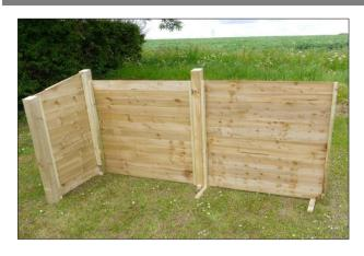
Rearrange the spacer blocks and offer up the next panel, aligning and attaching it as before.
