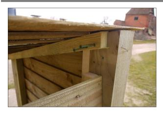
Secure the rear of the roof using shorter green screws as shown.
