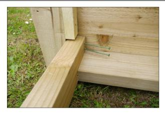
Attach the base to the end panel front post first, using 2 of the longer green screws.
