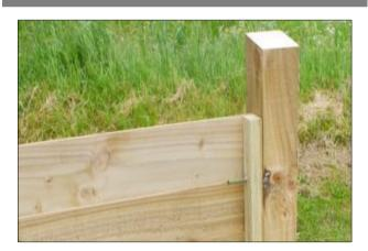
Align one of the longer posts (shorter for a reversed roof) with the other end of the back panel.
