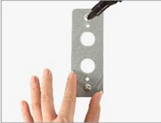
1. Mark the position of the hole
