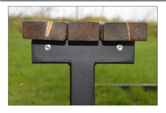
...and using the 70mm coach screws provided attach the seat panels to the leg-frame at both ends of the bench.
