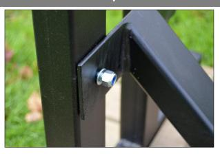
...and then offer up the the cross brace and loosely secure using a washer and a locknut for each of the two holes
