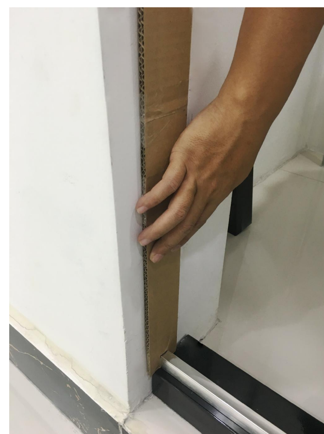
Insert template to bottom door guide.
