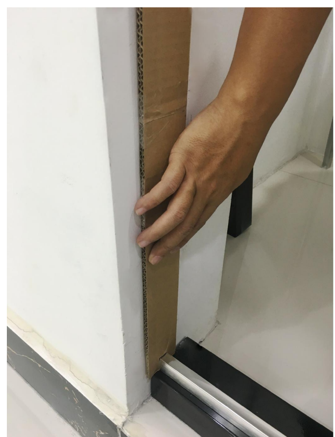
Insert template to bottom door guide.
