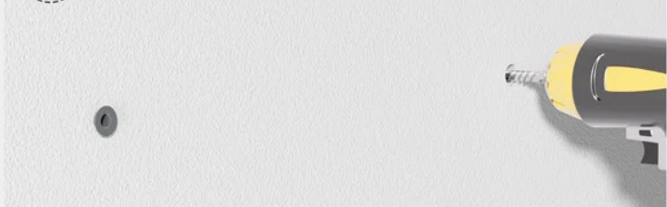
04 Drill holes in the wall
