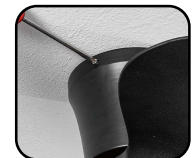
14 Tighten the fan, installation is done.
