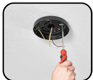
10 Tighten the base.
