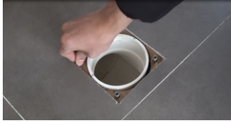
4. Put the screws into the holes
