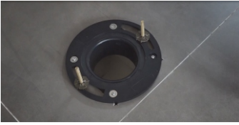
6. Install two long screws as below picture
