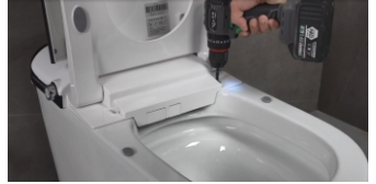
14. Install the screws on the toilet seat and put on the fixing
