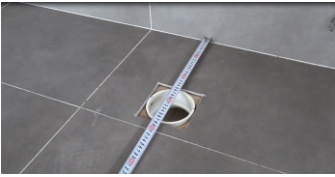
1. The confirmation of the installation environment, The measurement distance is 300mm or greater
