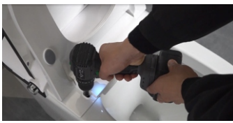
7. Unscrew the screws on the toilet seat
