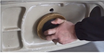
9. Turn over the toilet bowl and install the flange ring as below picture
