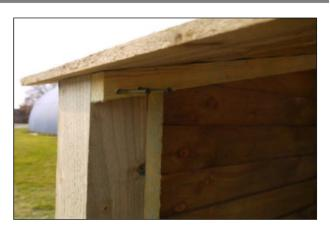
Check that the batten ends sit flush with the posts as shown. Now attach the roof to each end panel post with shorter green screws.
