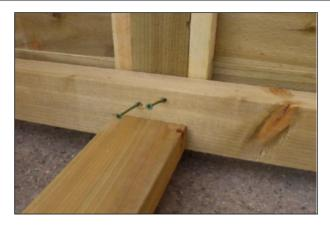
Using more of the longer screws now attach the base to the rear posts as shown.
