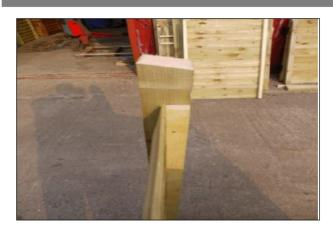
Attach the panel to the post by screwing through the batten using shorter green screws as before.
