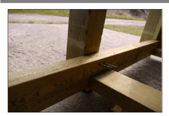
Check the positioning of the post within the guide marks once again before securing the bottom of the centre post with 2 of the longer green screws
