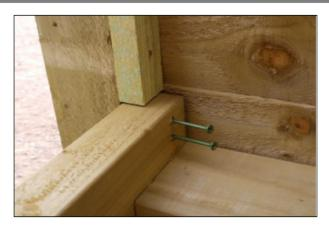
Attach the base to the end panel front post first, using 2 of the longer green screws and then secure the rear post in the same way.
