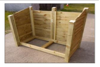
Slide the remaining end panel into place as shown above and attach it to the frame as you did with the first end panel with longer green screws into the front and rear posts. If you are fitting a kindling shelf, omit steps 12 -14 and attach the front posts before fitting the kindling shelf & lattice and then attaching the roof.
