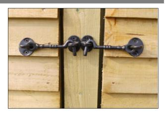
To fit the latch keeper plates, shut the door and hold the latch in the horizontal position. Now fit the keeper and mark its correct fixing position on the centre post using a pencil or bradawl before securing it in place using the screws provided.
