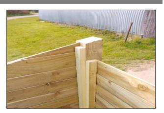
Using the shorter green screws provided, attach the batten on the back panel to the post of the end panel, ensuring that the batten remains vertically aligned to the post.
