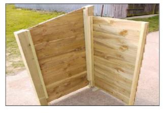
Arrange the 2 spacer blocks on the ground (the orientation is not critical), adjacent to the end panel as shown in the photo above. Now place a back panel on the blocks, at 90° to the end panel, aligning the 2 panels ready for fixing.
