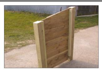
Stand the left hand end panel (or right hand for the reversed roof version) upright on a flat, level surface. Please note: The reversed roof model will have the highest point of the side panel at the front of the log store.
