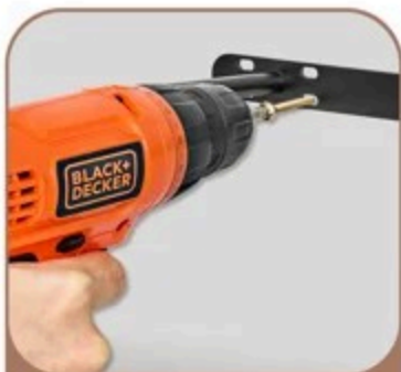
Attach Bracket to Wall
