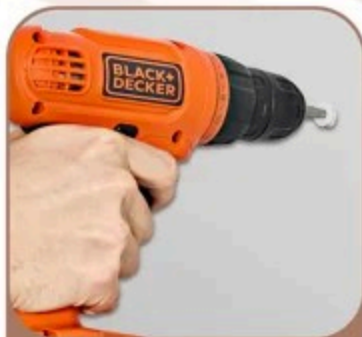
Drill Anchor into Wall
