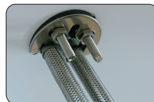
Put nuts on & tighten nuts
