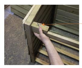
5. When attaching roof hinges ensure there is no gap, if needed pull down on roof and then attach hinge as shown in diagram
