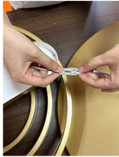
Step 2. Blue to blue line, brown to brown line insert connection
