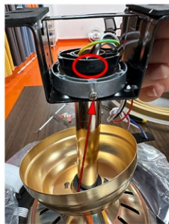
Step 14. Circle with arrow screws flat, button screws firmly fixed seat
