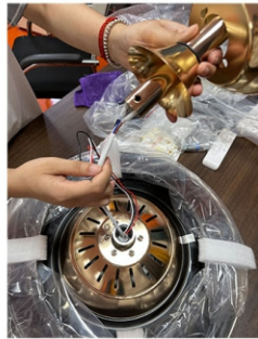
Step 8. Run all the wires through the boom
