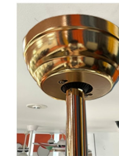
Step 17. Install the bell and horn cover, align the hole and rotate the bell to clamp firmly
