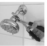
**Important:** Be sure to remove any old plumbers from shower pipe and in between shower pipe threads
