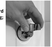
12. Screw smaller (nut) end of hose into shower diverter (ensure circular rubber washer is in place in hose); tighten with pliers
