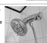
13. Screw shower brush head onto other end of hose (ensure circular rubber washer is in place in hose and remove plastic sheathing); tighten with pliers
