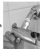
4. Cut two more 2-3 inch pieces of plumbers tape and wrap each piece around remaining two diverter threads
