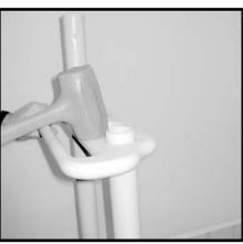
**Step 5:** Install towel rack/cup holder over the handrail posts with the towel rack to the outside of step, tap in place using the rubber mallet. Towel rack/cup holder may be positioned anywhere on the post.
