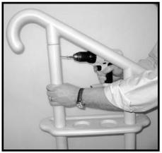
**Step 7:** Secure handrails using 1- # 10 x 1¼" screw into each post at pre-marked locations.
