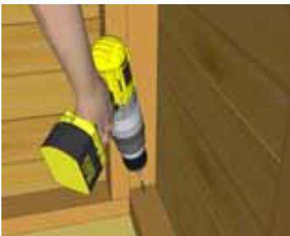
Angle screws into perimeter Floor Joists.
