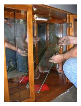
Slide the left side of the glass shelf into the case while rotating the glass flat.
