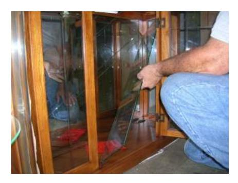
Insert right side of shelf it to the upper right corner of case with the plate groove side of shelf tilted downward.
