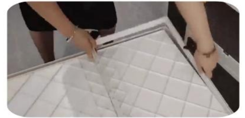
3.Remove the bottom fixing frame
