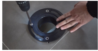
5. Put the flange ring into the drain outlet and install it
