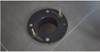
6. Install two long screws as below picture
