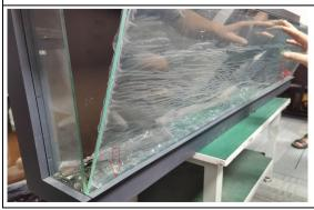
**Step 9:** Tear off the protective film both on the front and back of the large glass. **Note:** Before installing the metal pressure strip and the screws, you have to tear off the back protective film.
