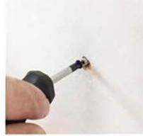
Step nine: Twist screw into expansion pipe and keep a little outside
