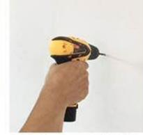
Step seven: Bore with drill of 6mm on the point of marks on the wall
