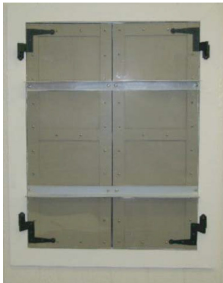
Two Storm Bars
