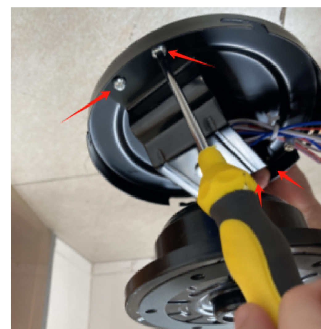
Hang the motor to the ceiling bracket
