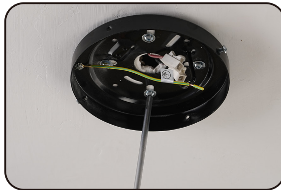
Step 5: Fix the mounting base to the ceiling with screws.
